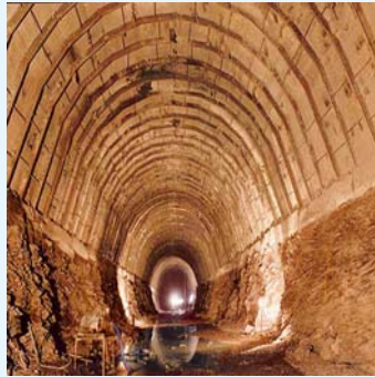
Tons Hydroelectric - MP
