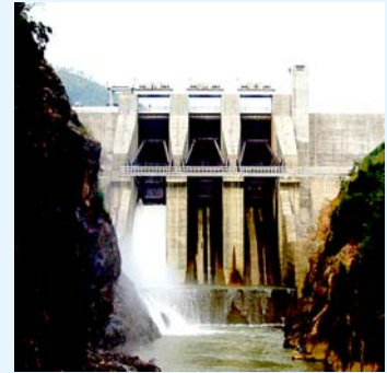
Water Supply Scheme - Shillong
