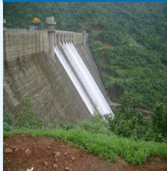
Ghatghar RCC Dam
